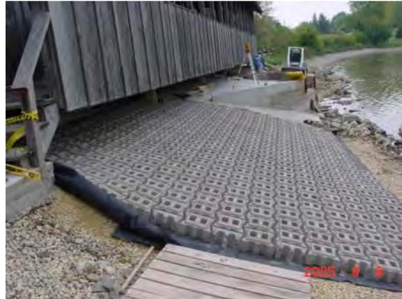
*Figure 8. Complete ArmorFlex Block installed*
