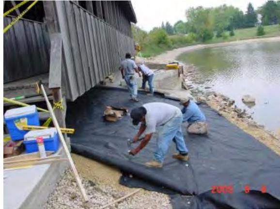
Figure 2. Installing the Geotextile
