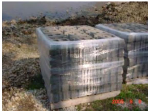
Figure 3. ArmorFlex on Pallets
