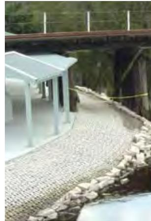
ArmorLoc® concrete interlocking blocks are specifically designed to control erosion. The ArmorLoc system provides easy and economical installation when equipment is not feasible or cannot be used due to confined or hard to reach areas. ArmorLoc is installed manually over site-specific filter fabric on a prepared surface. It improves the landscape and promotes drainage from the smallest erosion control job to the largest commercial project.
