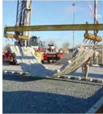
ArmorRoad® was developed in the field with input from contractors, construction managers and owners. The result is a flexible product that is efficient to install, aesthetically pleasing and able to withstand heavy traffic loads in harsh environments. ArmorRoad does not require the sand backfill typically required of standard pavers
