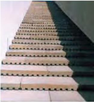
ArmorWedge® is a concrete step overlay protection system for embankment dams and spillways that are subject to high forces associated with overtopping flow. Researchers at Colorado State University assessed the stability of the blocks by comparing the downward (positive) forces of the block weight and the pressure of the flowing water to the uplift
