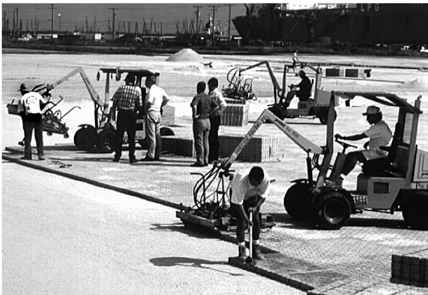
Figure 9. Mechanical installation equipment places concrete pavers rapidly.
