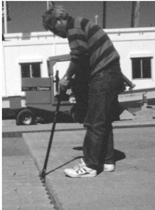
Figure 21. Once a few layers are removed by hand, then adjacent layers can be separated with a pry bar.
