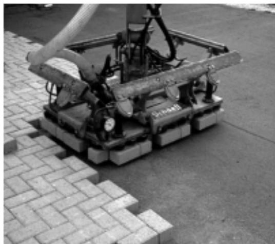
Figure 6. The vacuum head over the paver layer.
