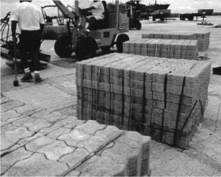
Figure 15. Spacing of cubes at the laying face is determined by how much area will be covered by each, as well as by the clearance required by the machine clamp. Orientation of the cubes follows the direction of paving.
