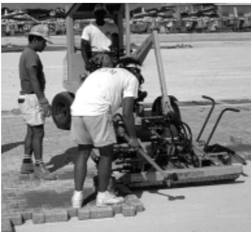
Figure 5. Motorized equipment with a hydraulic clamp.
