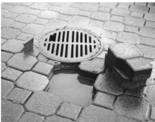
Figure 15. An absence of holes in the sides of this roof drain led to ponding.
