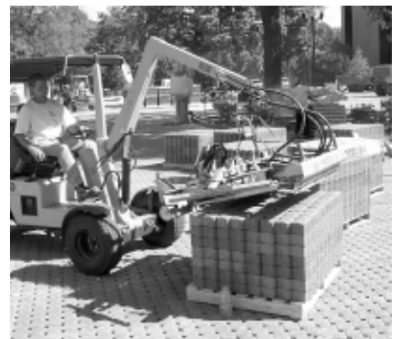
Figure 1. Mechanical installation of interlocking concrete pavements (left) and permeable units (right) is seeing increased use in industrial, port, and commercial paving projects to increase efficiency and safety.
