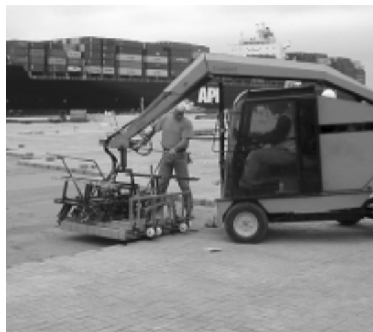
Figure 1. Mechanical installation of interlocking concrete pavements (left) and permeable units (right) is seeing increased use in industrial, port, and commercial paving projects to increase efficiency and safety.
