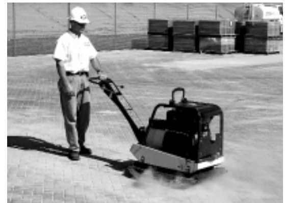
Figure 12. Final compaction should consolidate the sand in the joints of the concrete pavers.
