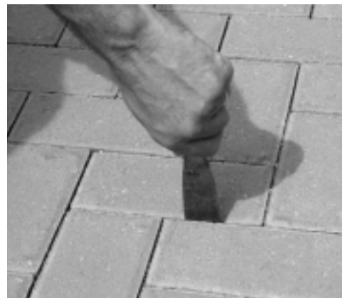
Figure 13. A simple test with a putty knife checks consolidation of the joint sand.
