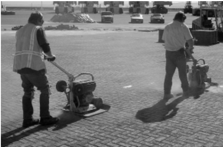
Figure 9. Initial compaction sets the concrete pavers into the bedding sand.
