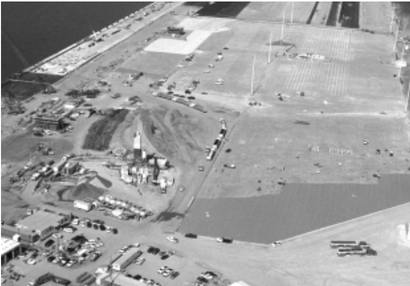
Figure 14. The Port of Oakland, California, is the largest mechanically installed project in the western hemisphere at 4.7 million sf (470,000 m 2 ).
