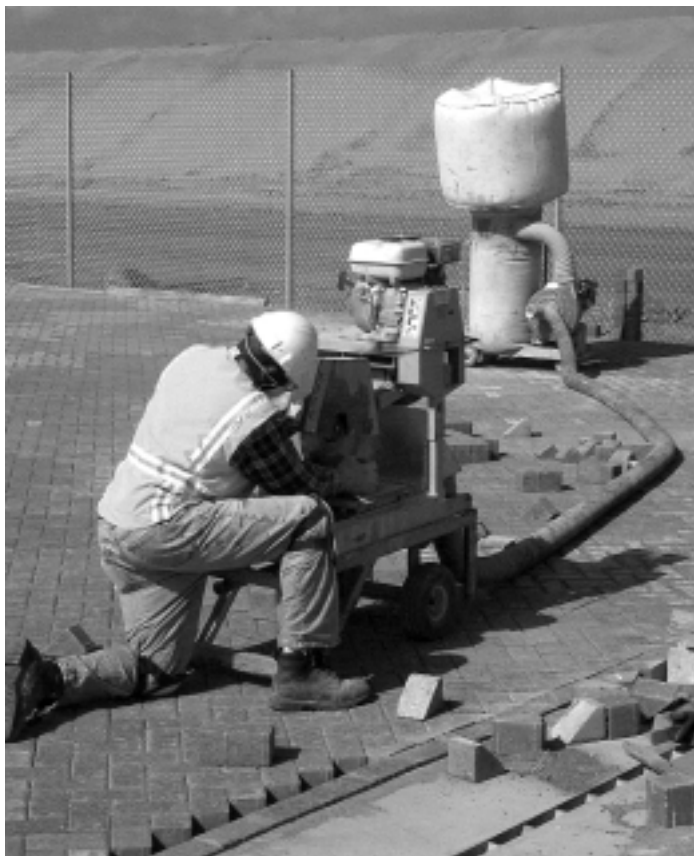
Figure 8. Edge pavers are saw cut to fit against a drainage inlet.
