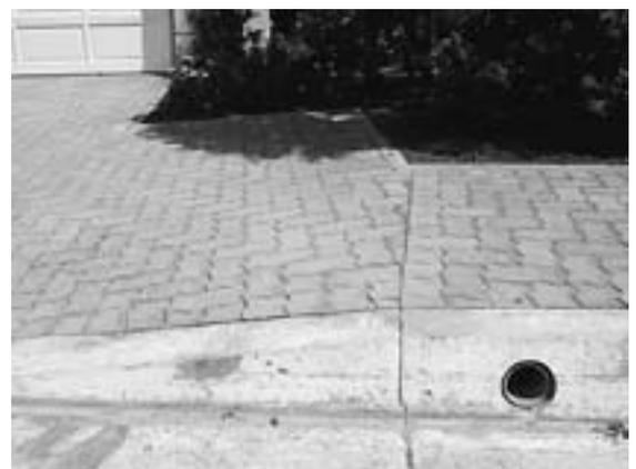
Figure 3. Ramp pavers changing angle.
